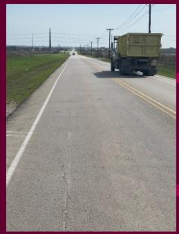
City Portion Minimal Preventative Maintenance Original Surface (18 years old) Solid with a Few Isolated Failures County Portion Regular Prev Maint (Crack Sealing) Asphalt Overlay in 2016
