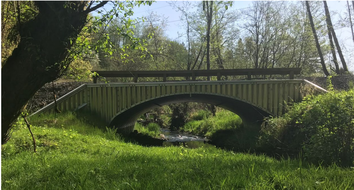
Aluminum Structural Plate Headwall/Wingwalls
