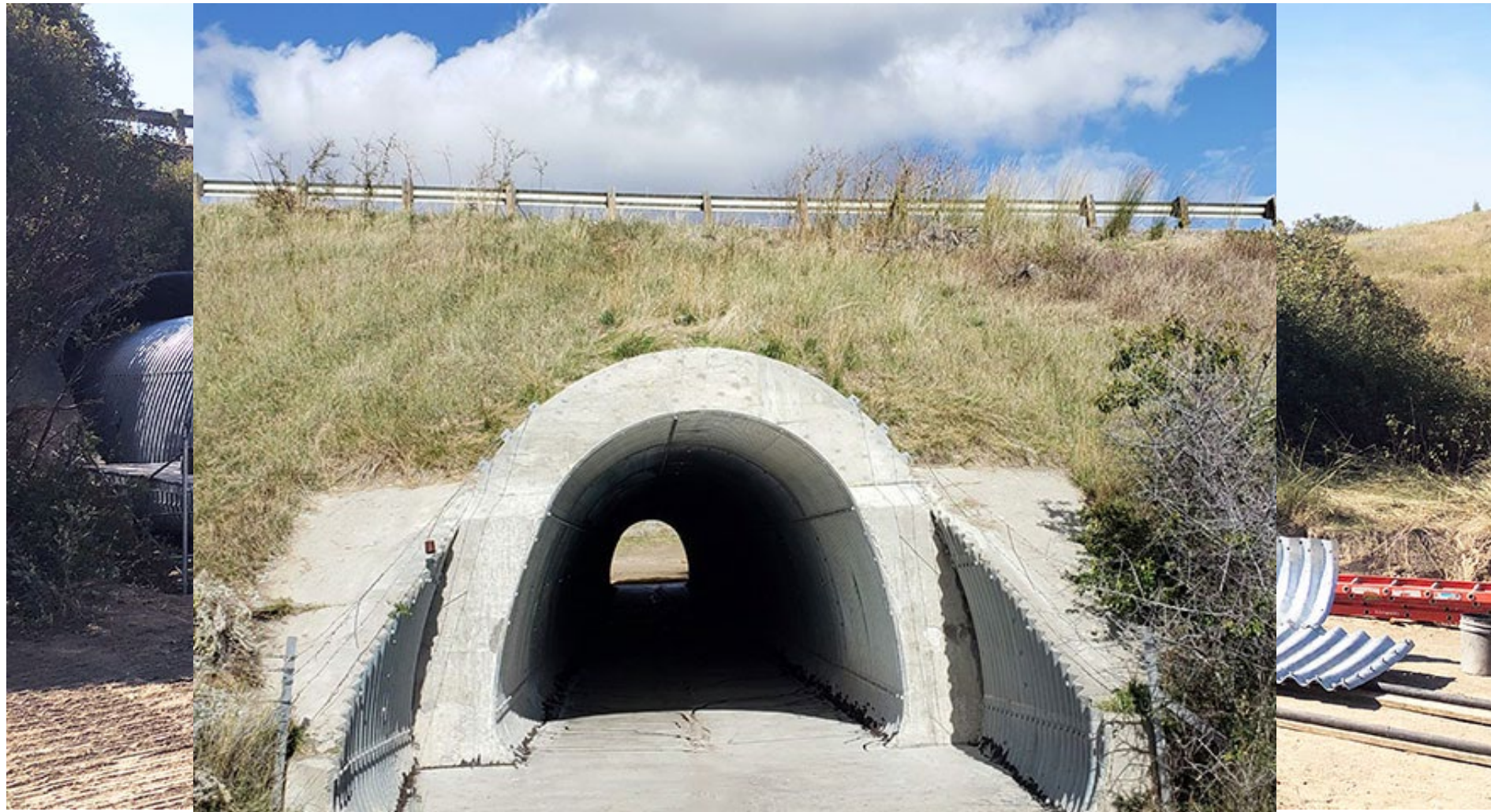
2020 NSCPA Project of the Year - Multiplate - I-94 Montana DOT – Reline 11'-4" x 10'-3" Underpass
