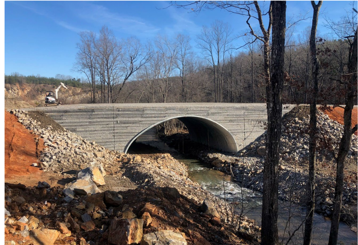
60'-4" Span X 22'-8" Rise 2-Radius Arch BridgeCor
