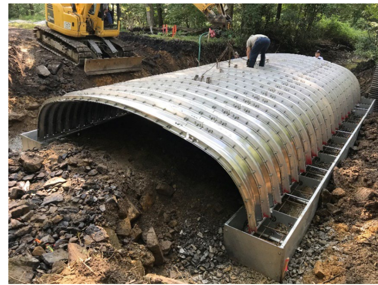
Steel EXPRESS Foundations
