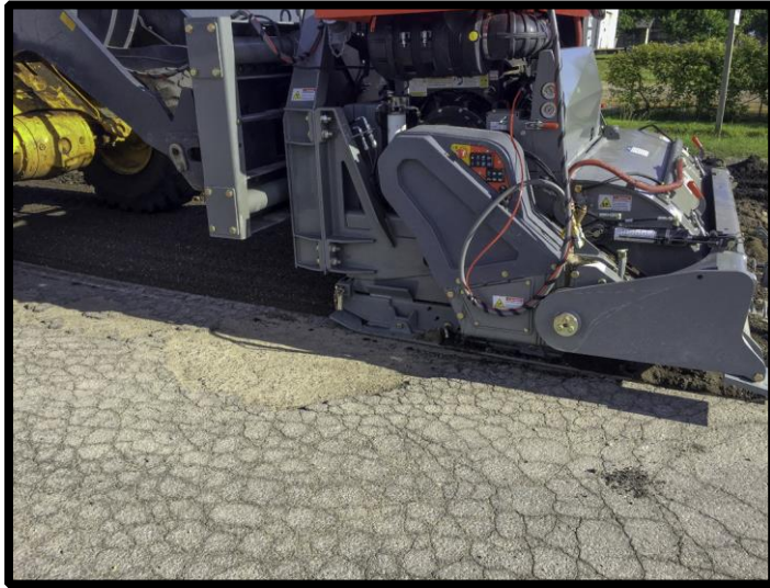
Asphalt Zipper reclaiming badly alligatored asphalt
