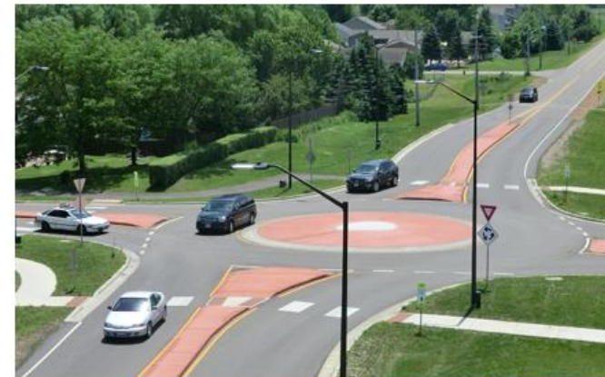
Example of a single-lane roundabout. Source: FHWA
