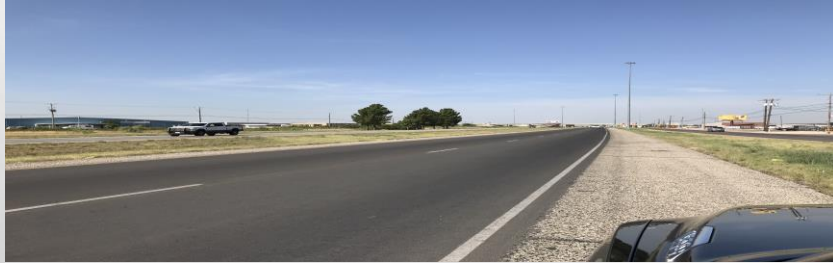
Micro-surfacing - $3.5-$4.5 per Square Yard = $56,320/Mile
