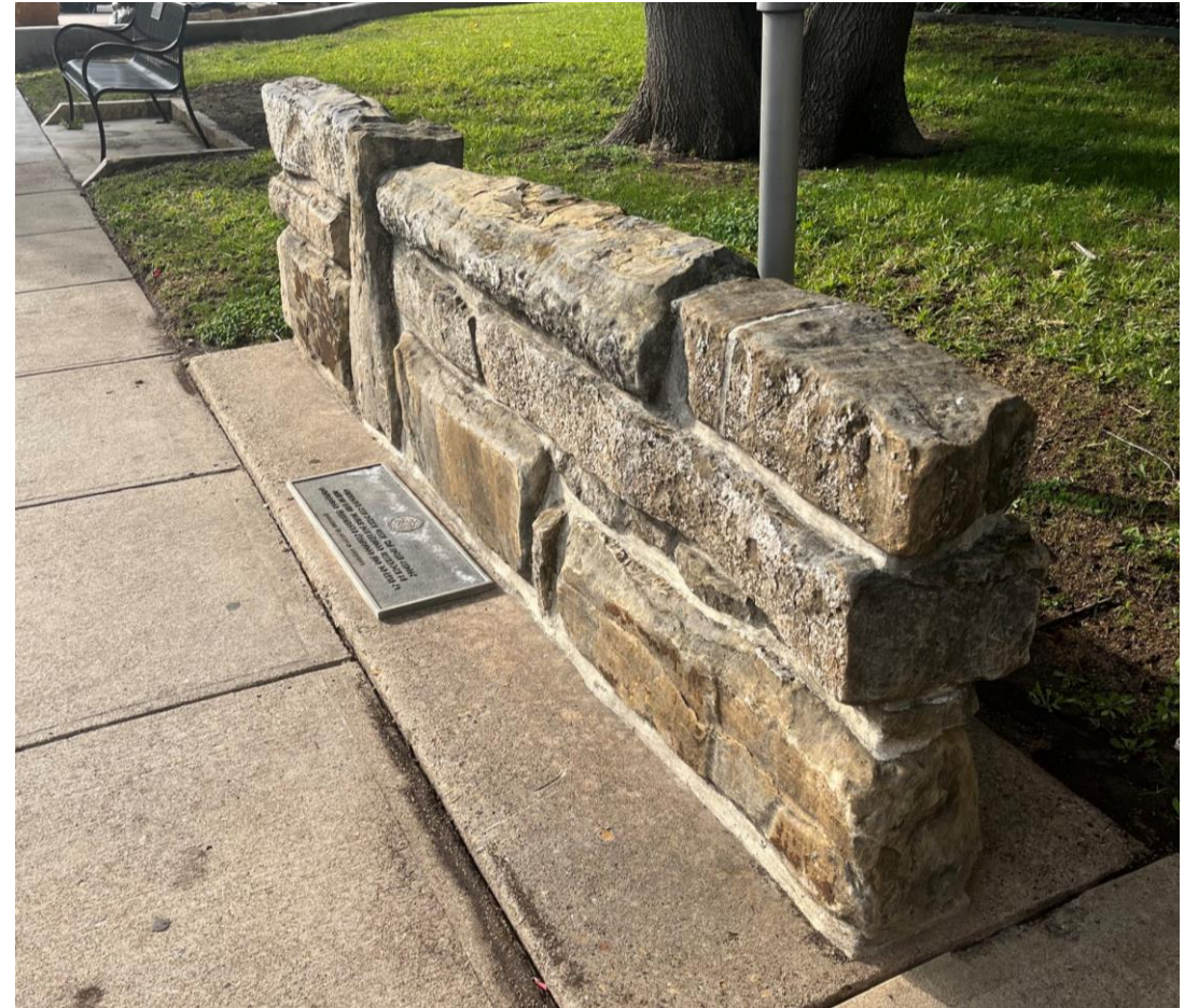
Portion of the rock wall
