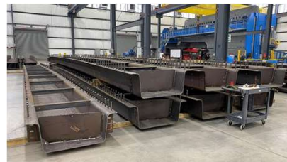
FINISH WELD STATION
