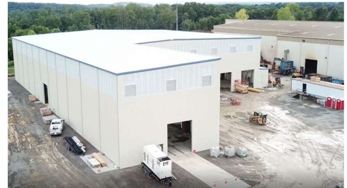
PURPOSE BUILT PRESS BRAKE TUB GIRDER FACILITY
