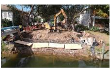
Birch Road Bridge – Construction of bridge abutment
