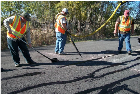
Men crack sealing a roadway in central Texas
